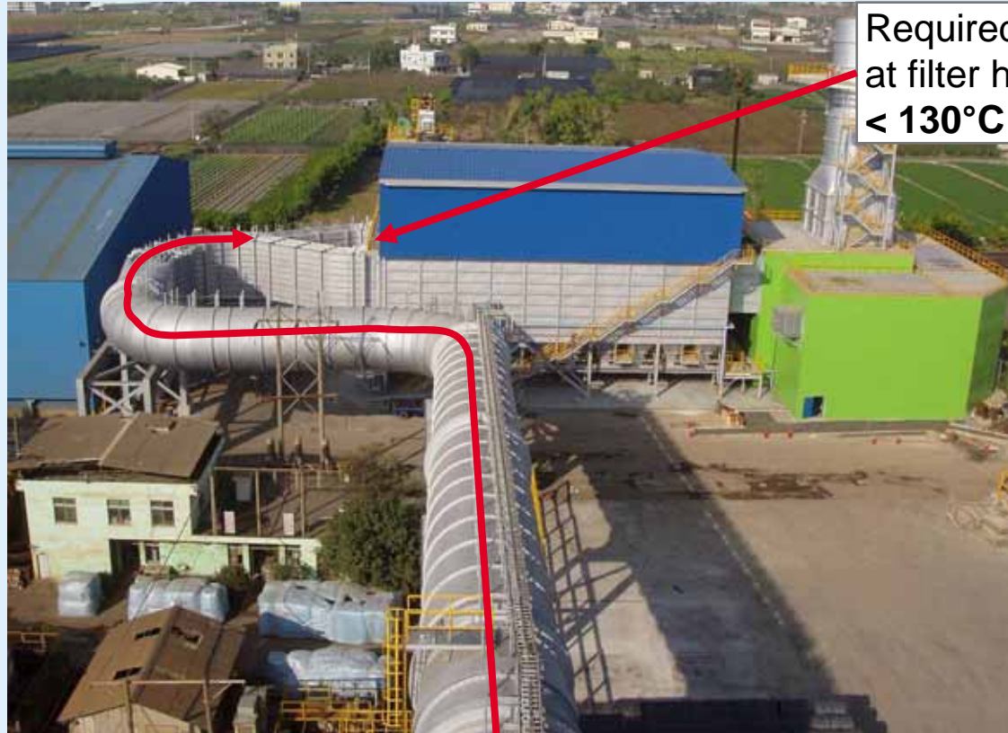
EAF off-gas duct to filterhouse
